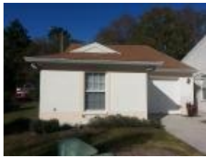
E & R House Done
